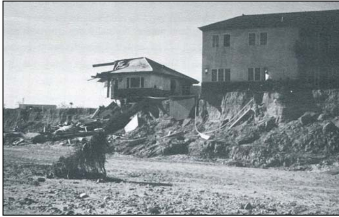
Figure 5. Damaged Office Building on the Rillito River
