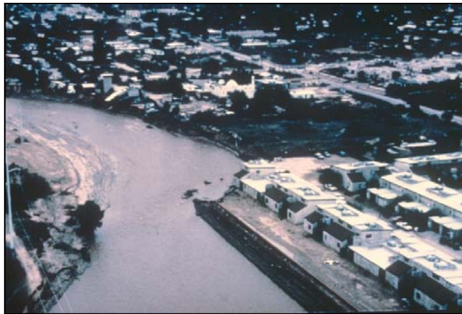
Figure 20. Comparison Soil-Cement and Unprotected Banks on Rillito River, Tucson, Arizona
