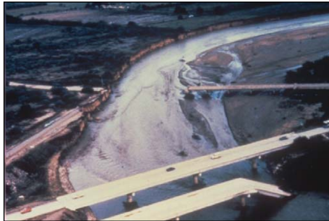
Figure 19. Collapse of I-19 Bridge south of Tucson, Arizona
