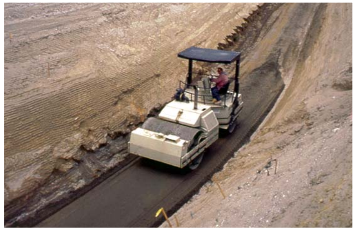
Vibratory compactor shown compacting soil-cement lift.
